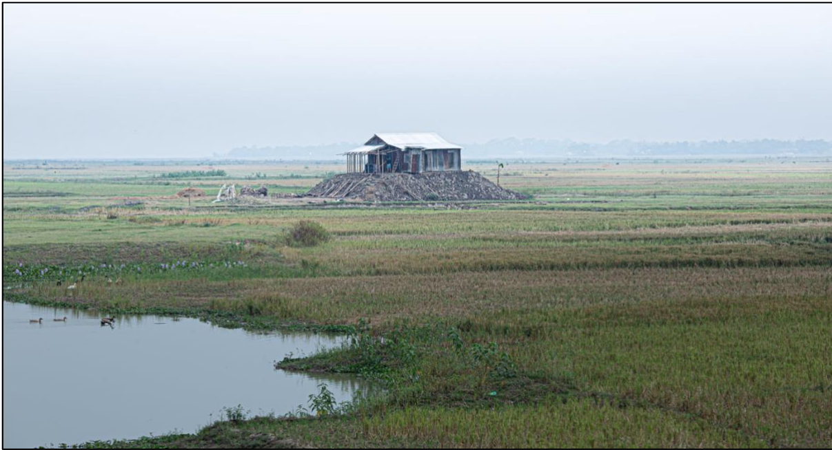
Figure 2. People elevate their homesteads to protect against annual flooding in the haor region. source: author.
