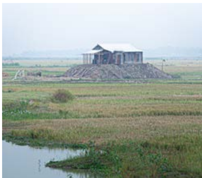
Figure 2. People elevate their homesteads to protect Against annual, routine flooding in the Haor region. Source: author.
